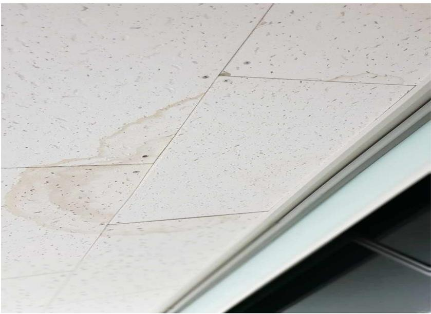
A photograph showing significant water damage on a white, textured ceiling. The damage is characterized by large, irregular brown stains that spread across several ceiling tiles. The tiles are separated by dark grid lines. In the bottom right corner, a portion of a light blue door frame is visible.                                                                         |                     |
